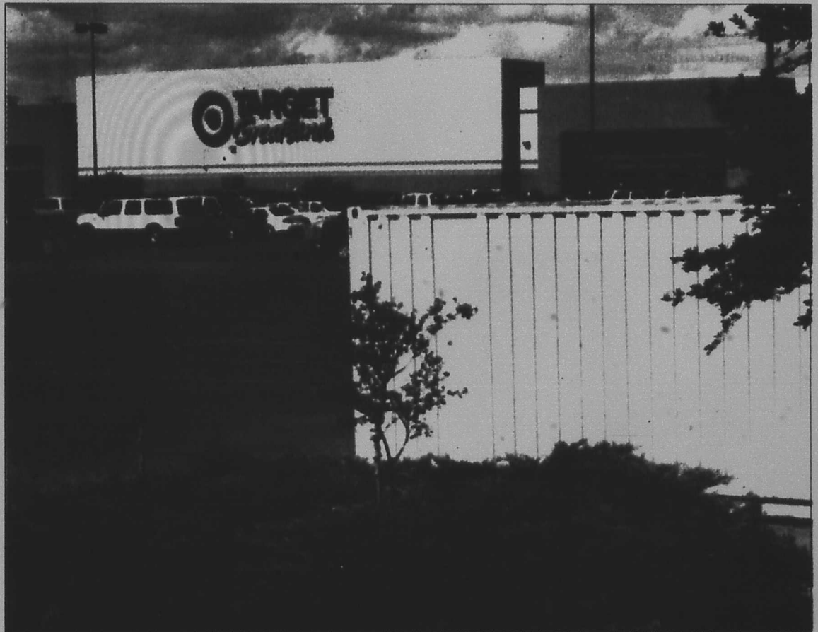
Cuate Santos/Laredo Morning Times CHANGES: Containers with tools and supplies sit outside Target in the North Creek shopping center Wednesday in preparation for the discounter's remodeling project.
